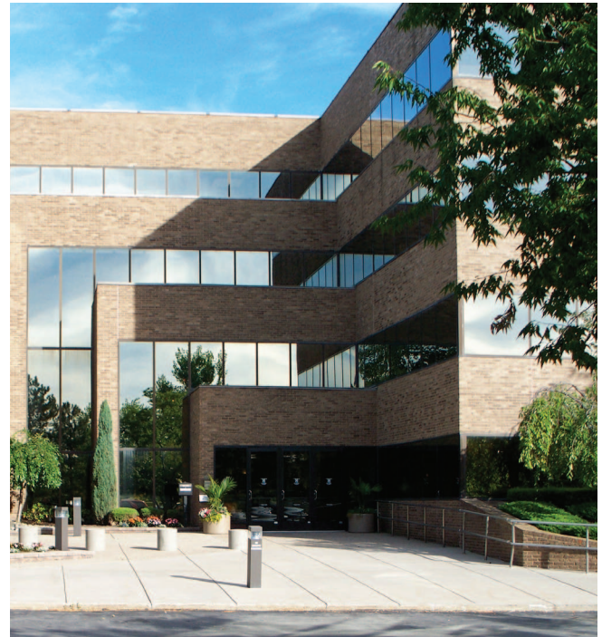
Data Center located in Amherst, NY
